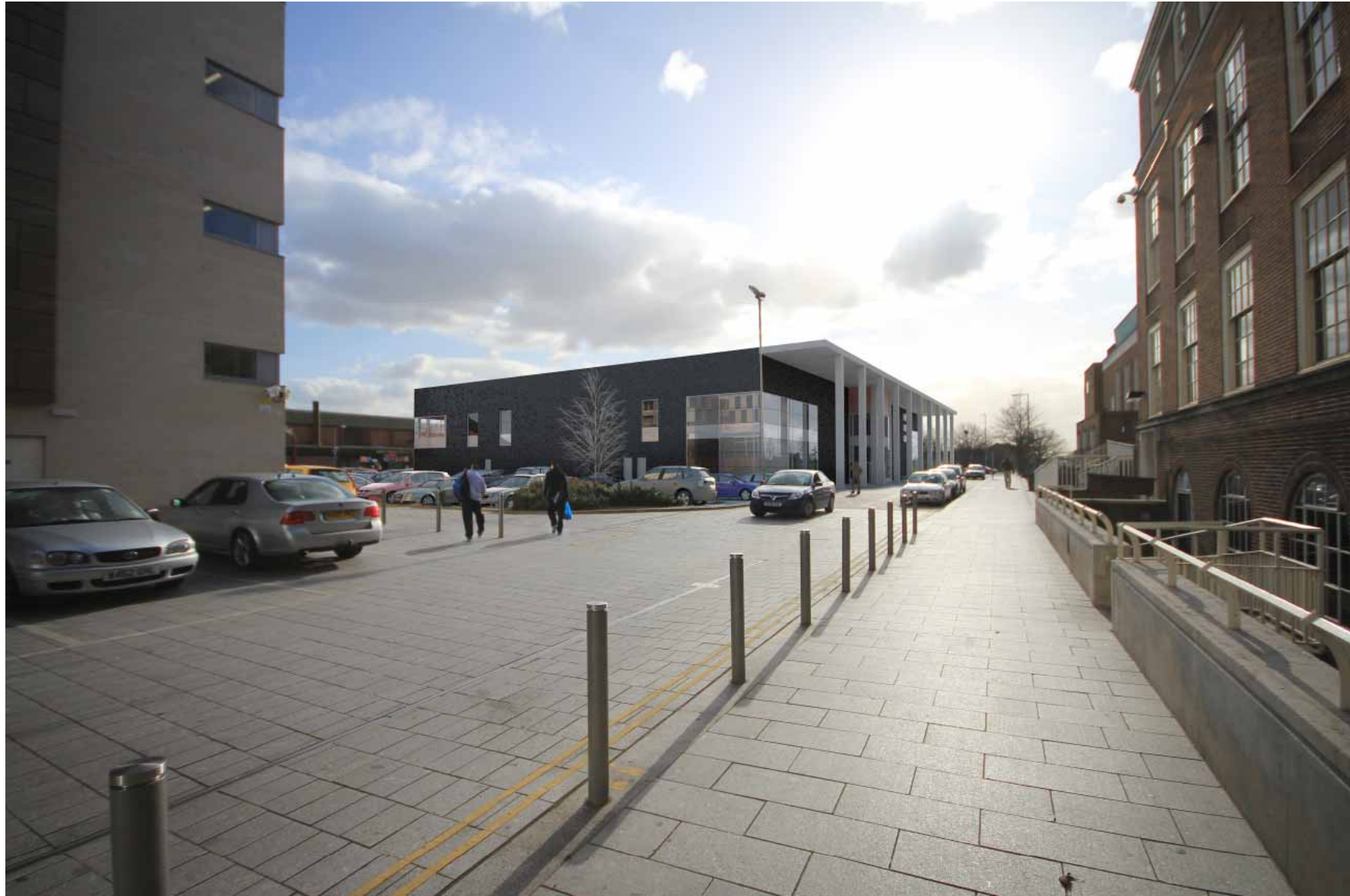
EXTERIOR VISUALISATION FROM THE TOWN SQUARE – SOUTH WEST CORNER
